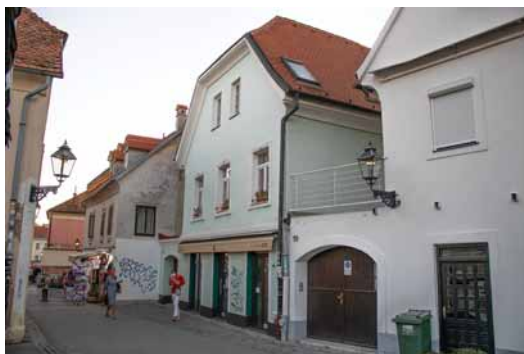
Fig. 6 Opatovina 17, Gregurić House (photo by M. F. Pavković)
