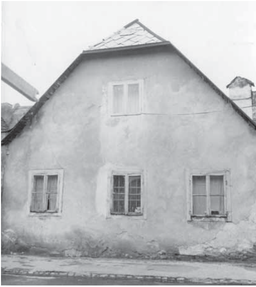
Fig. 2 Opatovina 21, house, eastern (street) front (MK-UZKB-KOZ, photo by Lj. Krtelj, 1965, inv. ref. no. 9503)
